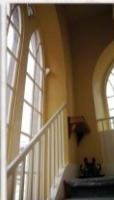
Interior photograph of stairwell and vestibule, noting the lead covered stairs, added so convicts would not ruin the woodwork
